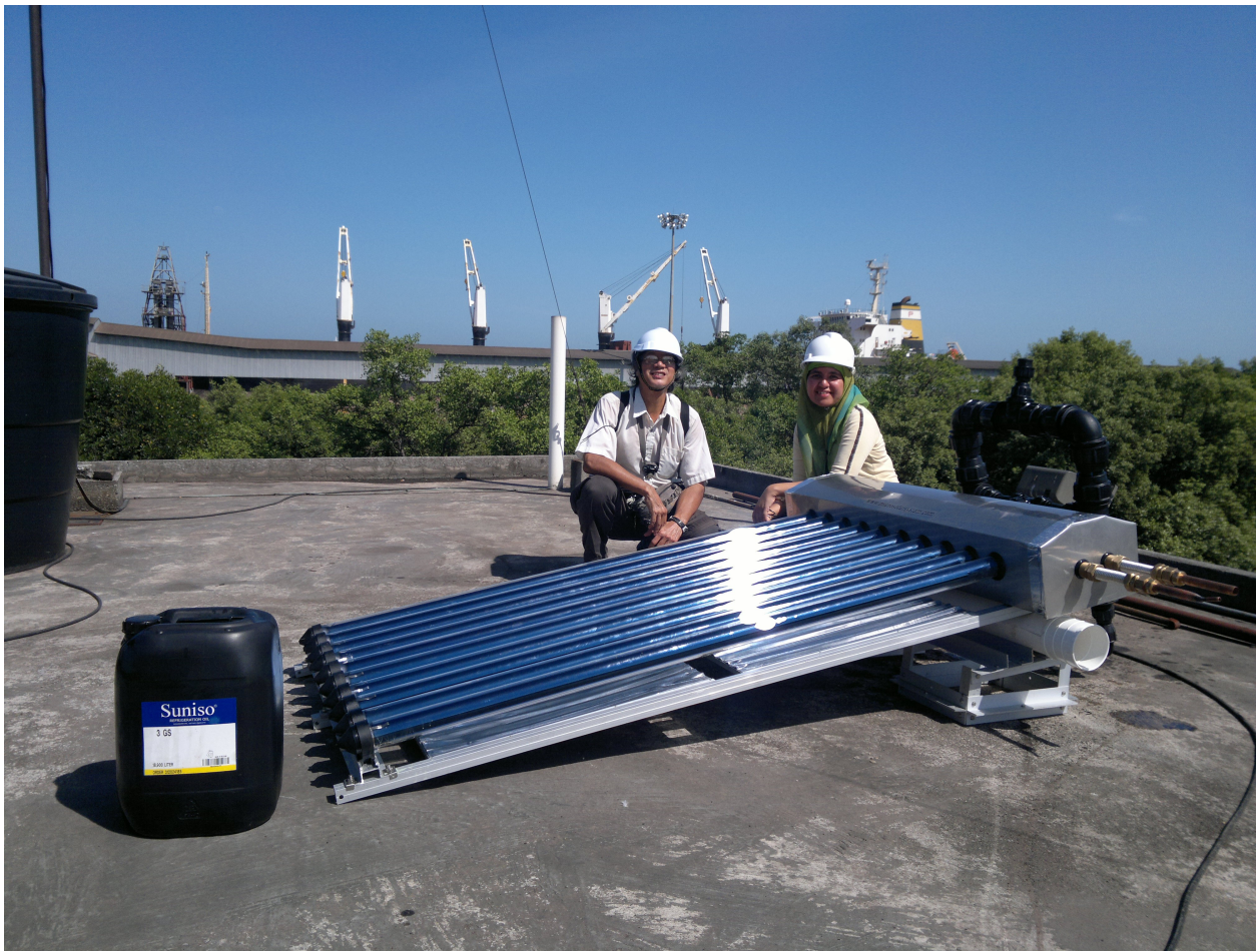
Siang and Azrina with the Microsolar Manifold unit of Alam Dingin's Solar Air Conditioner on the roof of the Bomba Tower at North Port, Port Kelang, Selangor, Malaysia. June 2013
