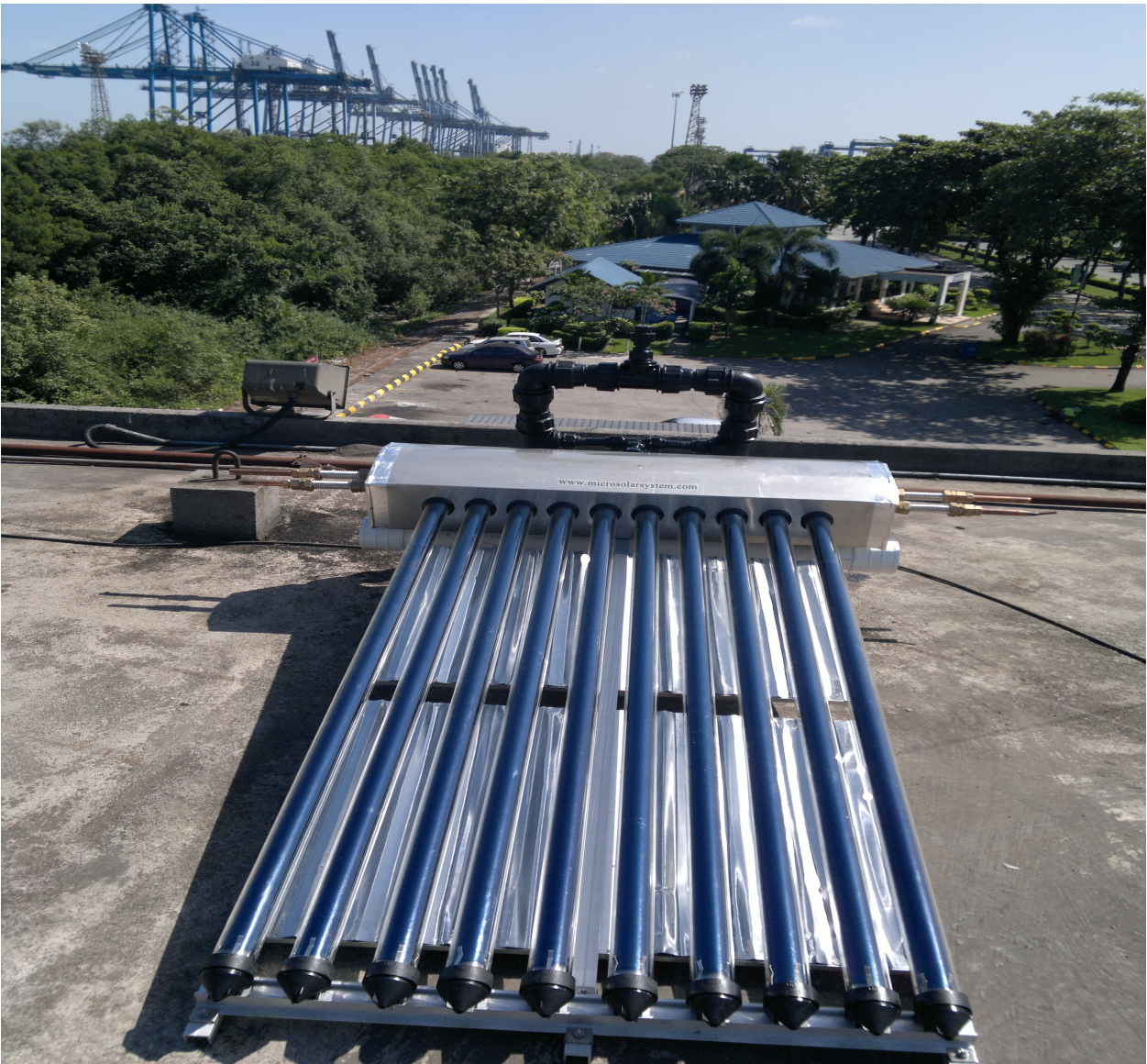
Microsolar Manifold unit of Solar Dingin Solar Air Conditioner installed at North Port, Port Kelang, Selangor, Malaysia.
