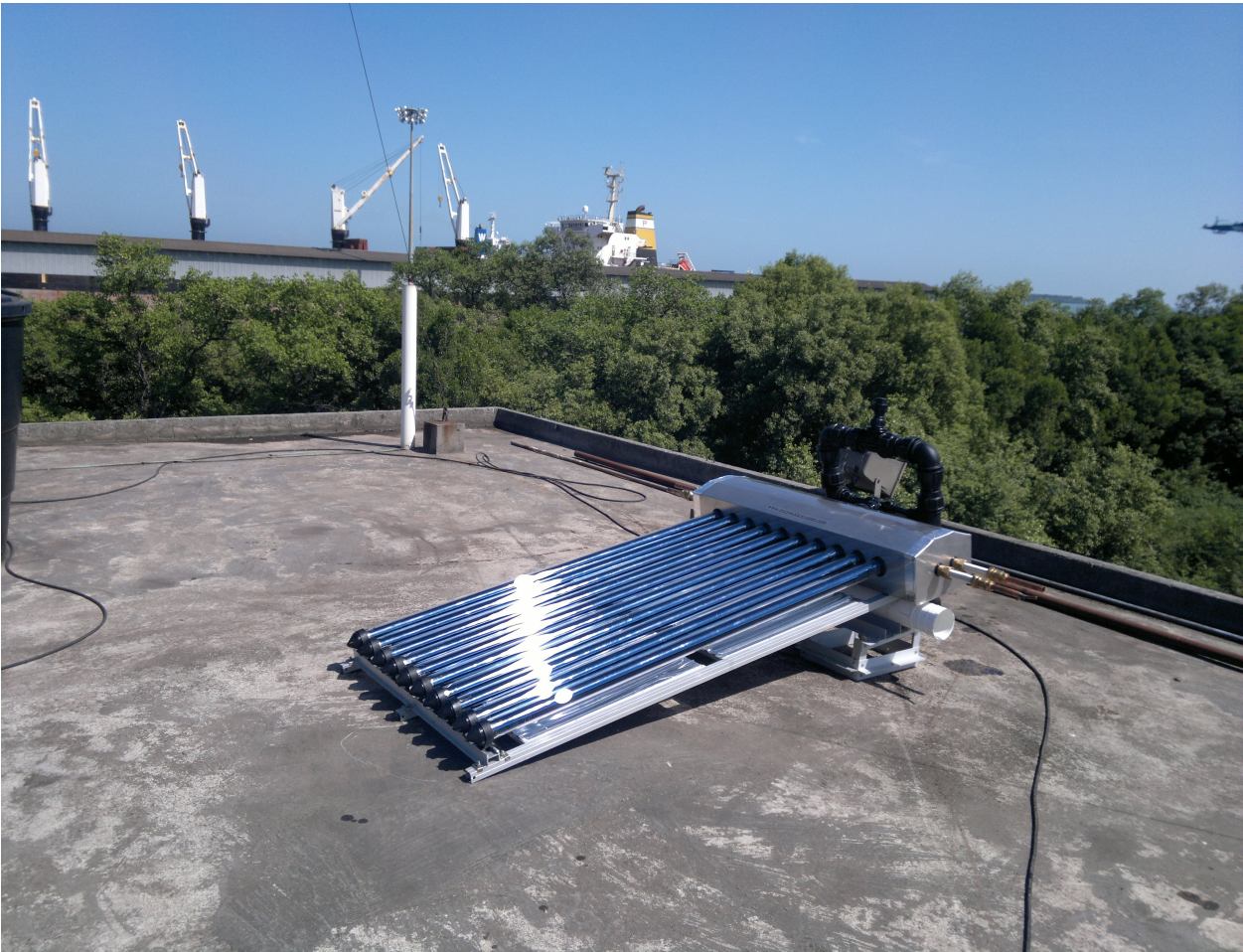
Microsolar Manifold unit of Solar Dingin's Solar Air Conditioner installed on Bomba Tower North Port with the Container wharves in background
