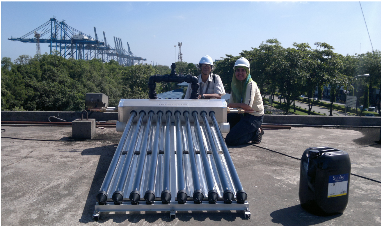
Siang of Microsolar and Azrina of Solar Dingin with the Alam Dingin Solar Air Conditioner's Microsolar Manifold on the roof of the Bomba Tower at North Port, Port Kelang, Selangor, Malaysia.
