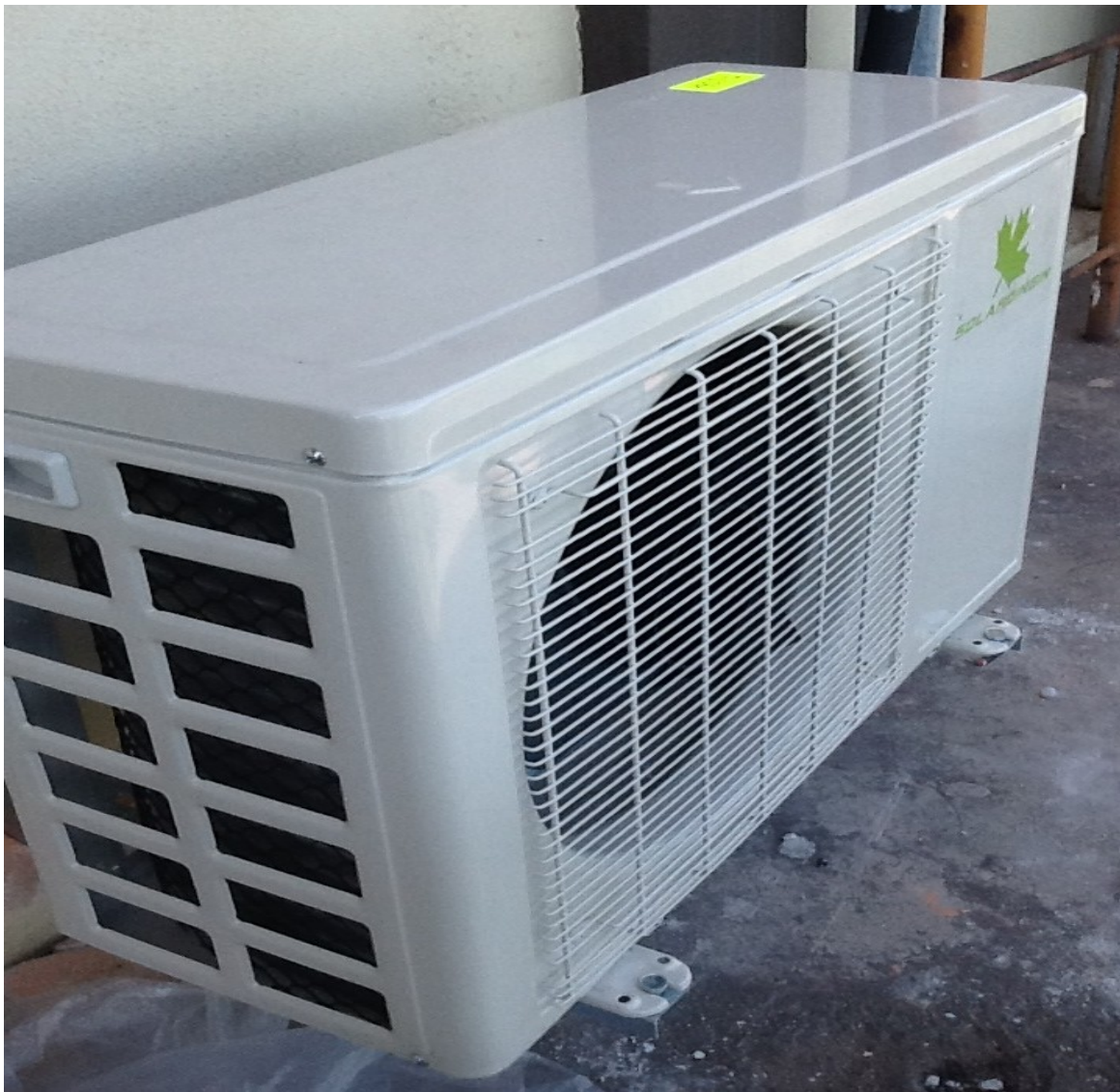
Solar Dingin Solar Air Conditioner Outdoor Unit completed installation at North Port, Port Kelang, Selangor, Malaysia. June 2013
