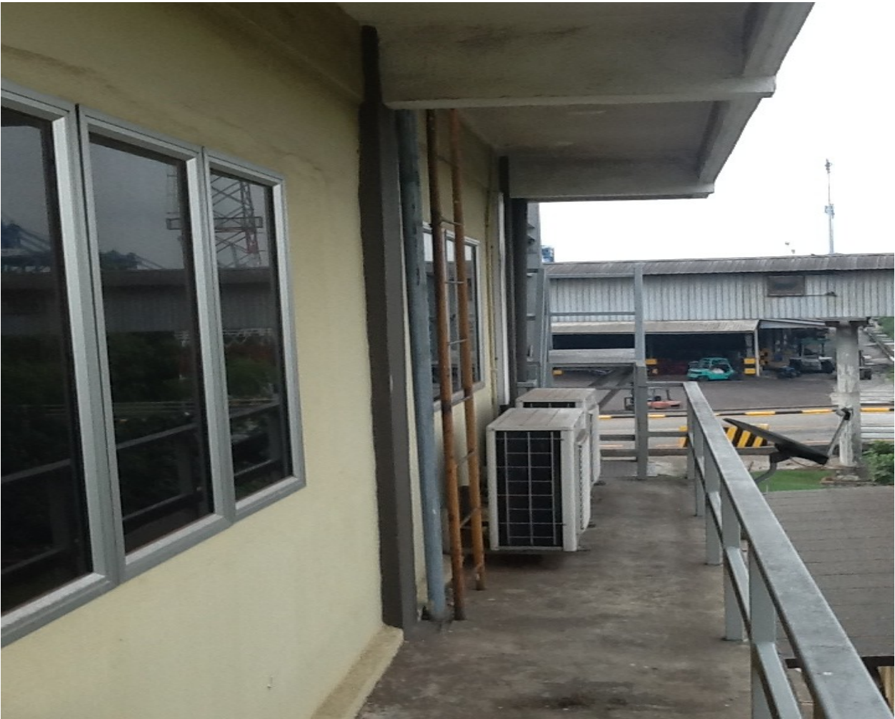
Installation site at Bomba Tower, North Port, before installation of Solar Dingin Solar Air Condioner
