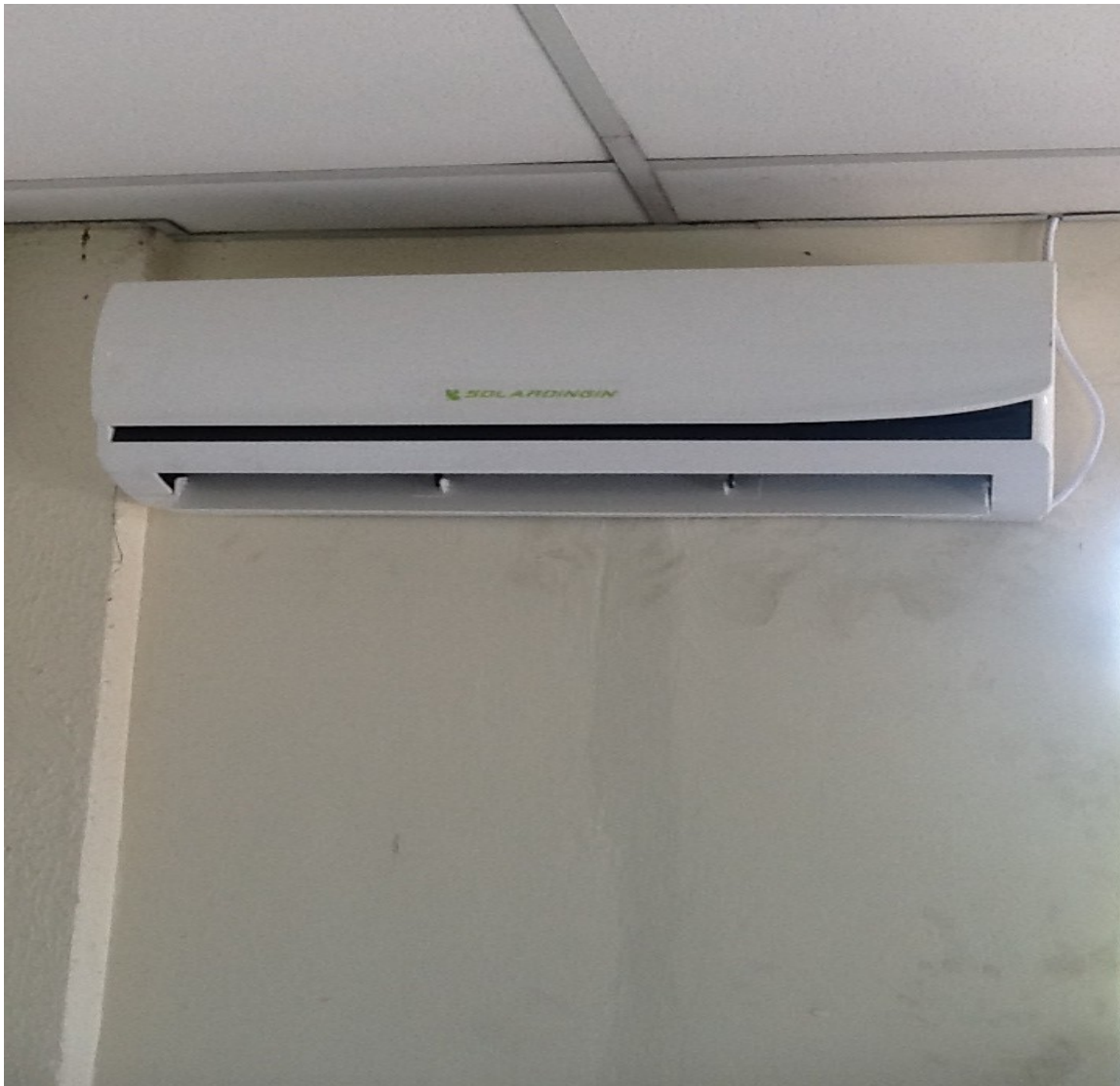
Solar Dingin Solar Air Conditioner 1.5 hp Indoor Unit completed installation inside Bomba offices at North Port, Port Kelang, Selangor, Malaysia.
