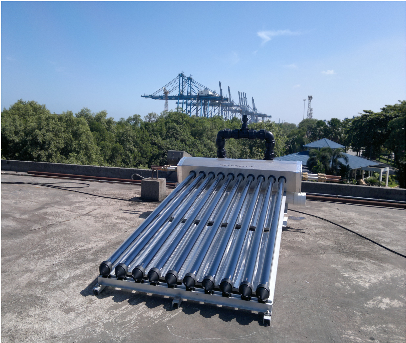
Microsolar Manifold unit of Solar Dingin Air Conditioner installed at North Port, Port Kelang, Selangor, Malaysia. June 2013
